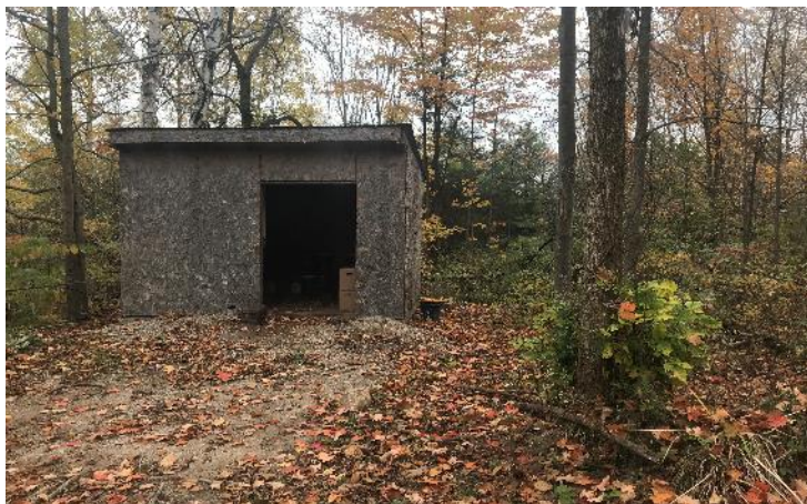
Image 4: CBM Lanci Stage 2, area of disturbance, abandoned shed, facing north.
