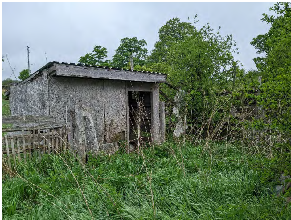
Photo 2 Abandoned shed structures on Site surrounded by grasses and shrubs.
