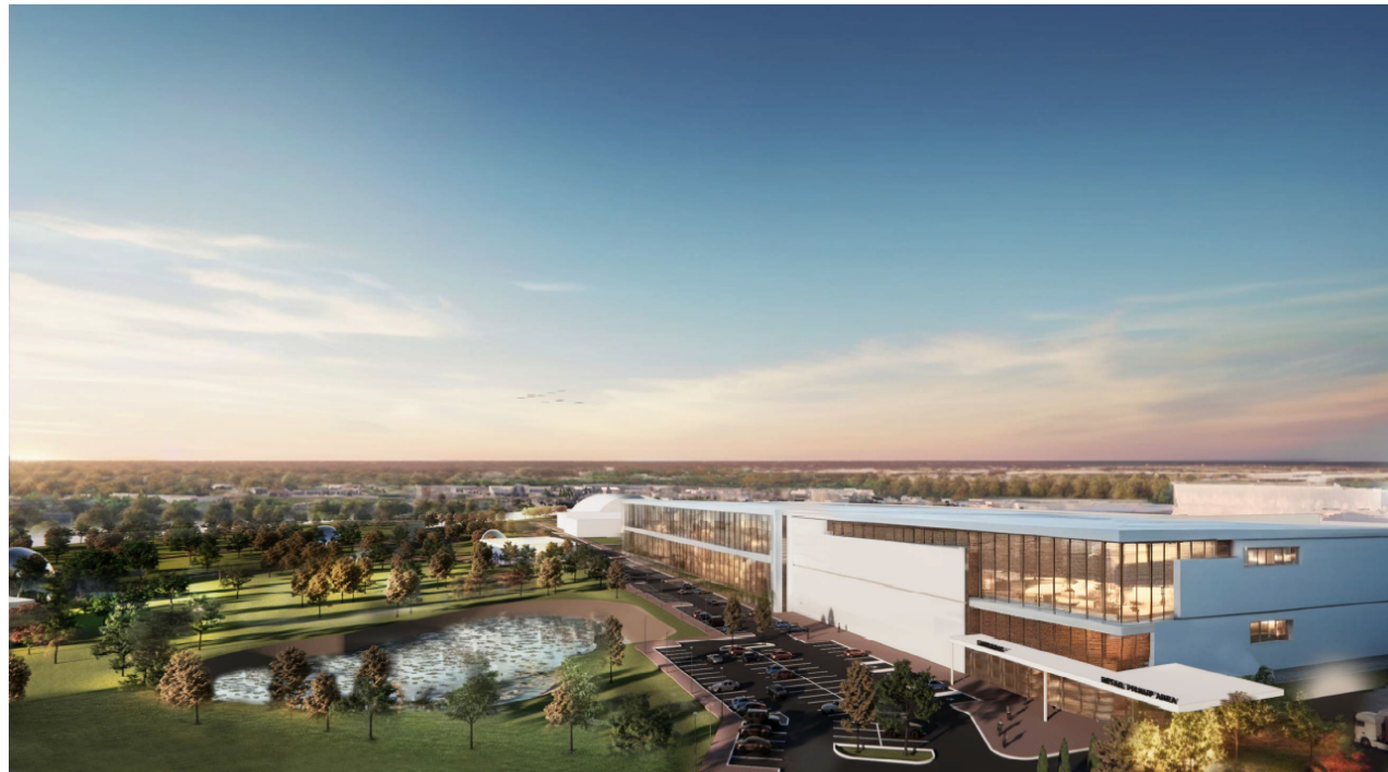
AERIAL VIEW LOOKING WEST
