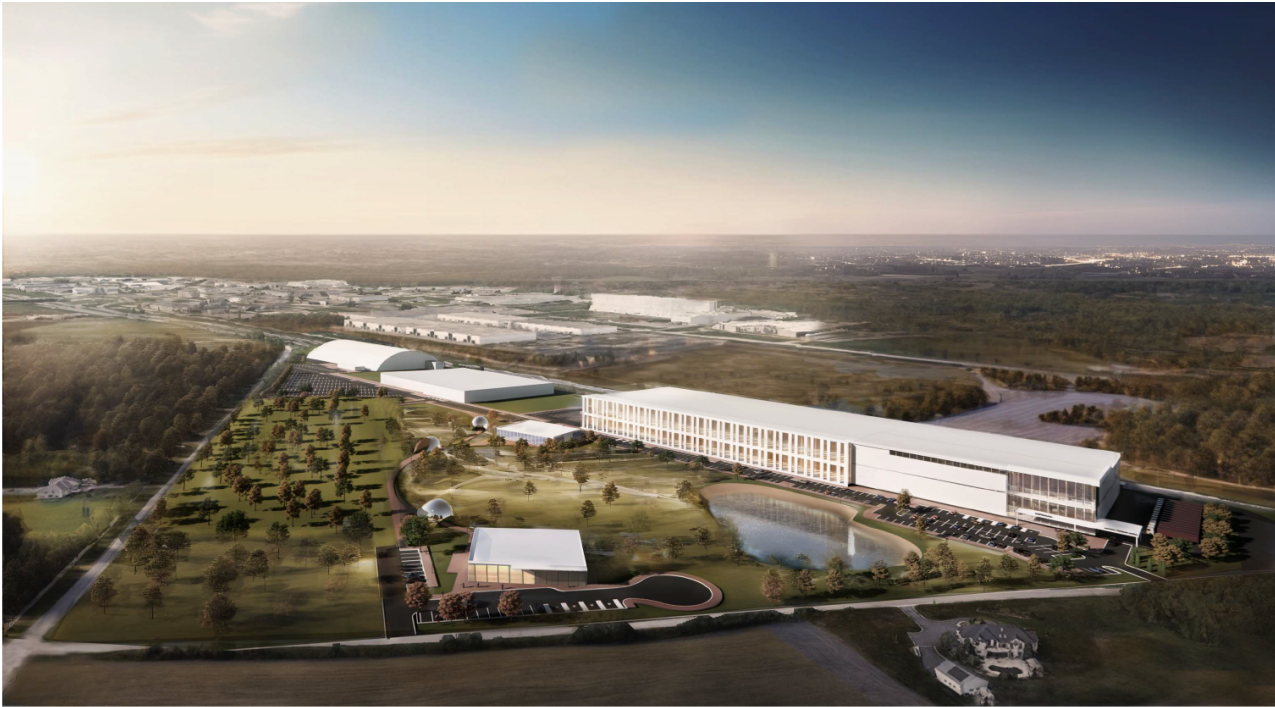
AERIAL VIEW LOOKING NORTH
