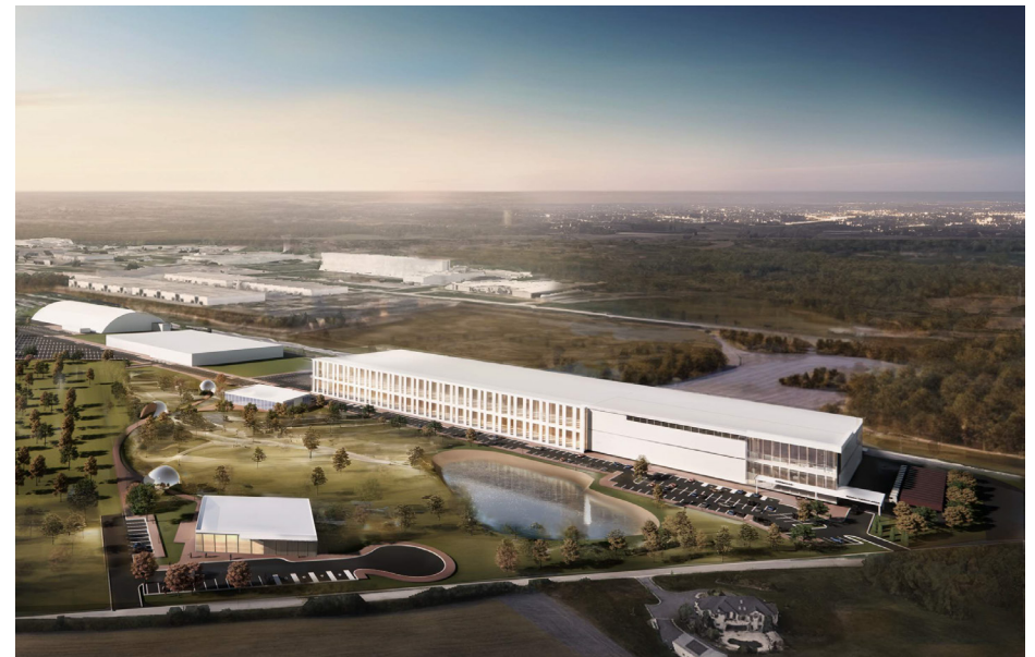
Aerial View Looking North
