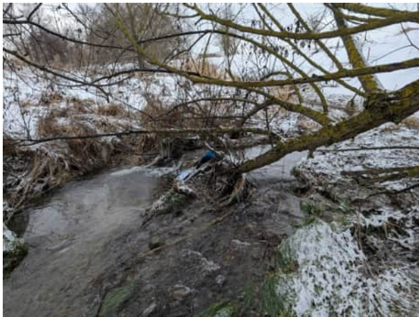
Photograph 15 Location 12 Reach FCT-2
