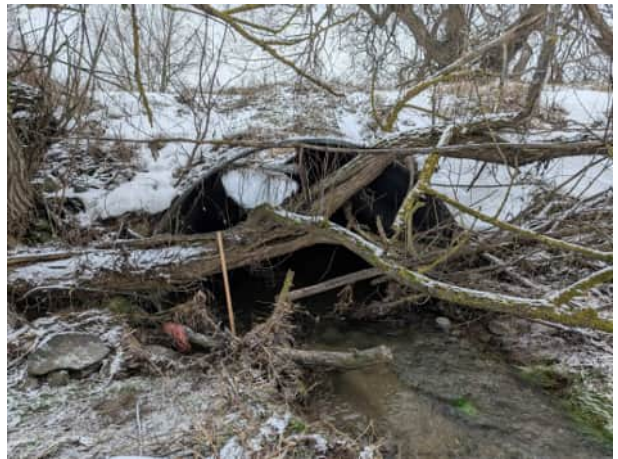
Photograph 16 Location 12 Reach FCT-2
