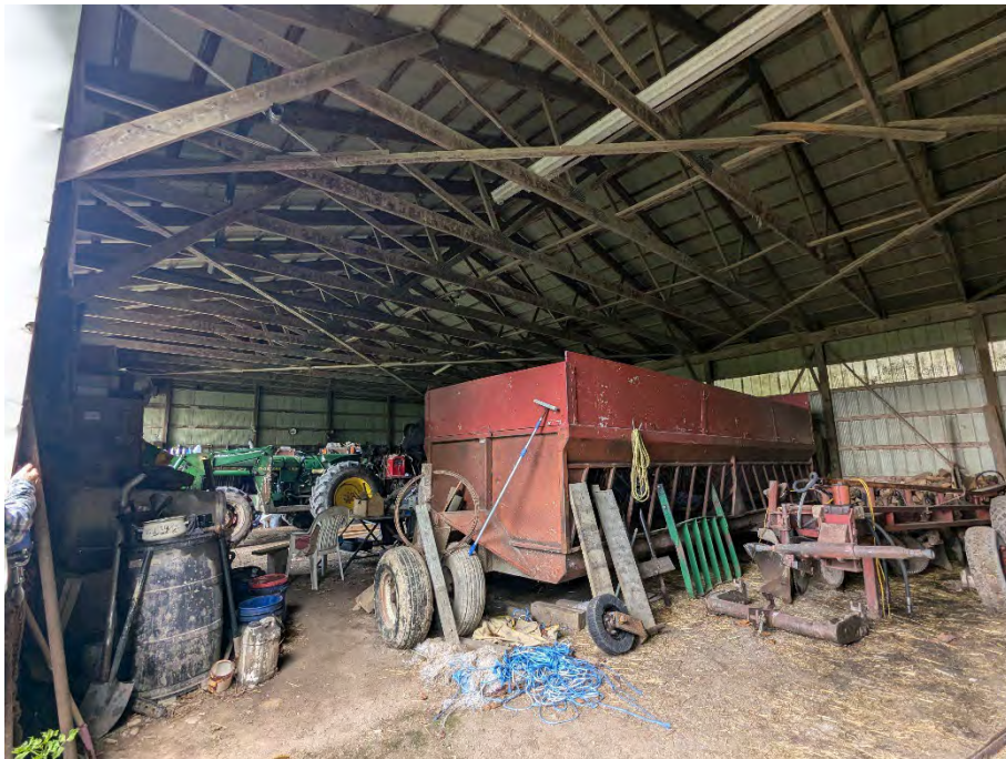
Photograph J14 – Interior of maintenance garage, showing two drums, looking northwest.
