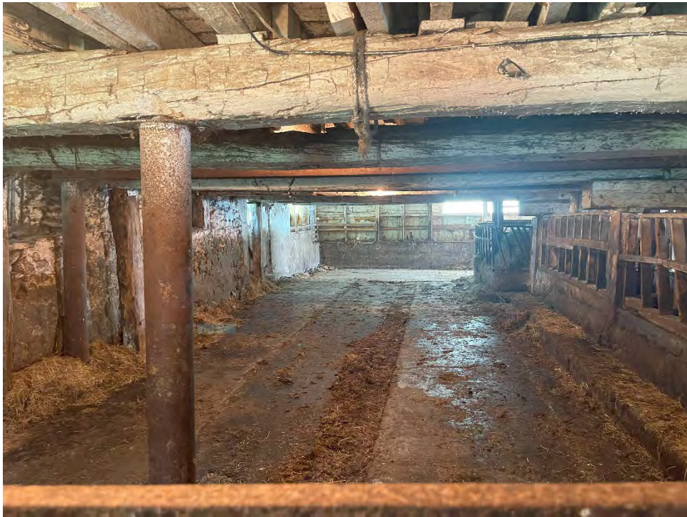
Photograph J7 – Lower level of barn, looking east.
