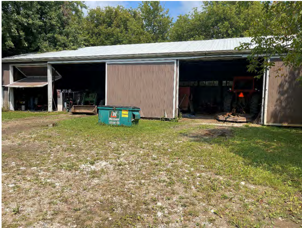
Photograph J11 – Maintenance garage, looking north.
