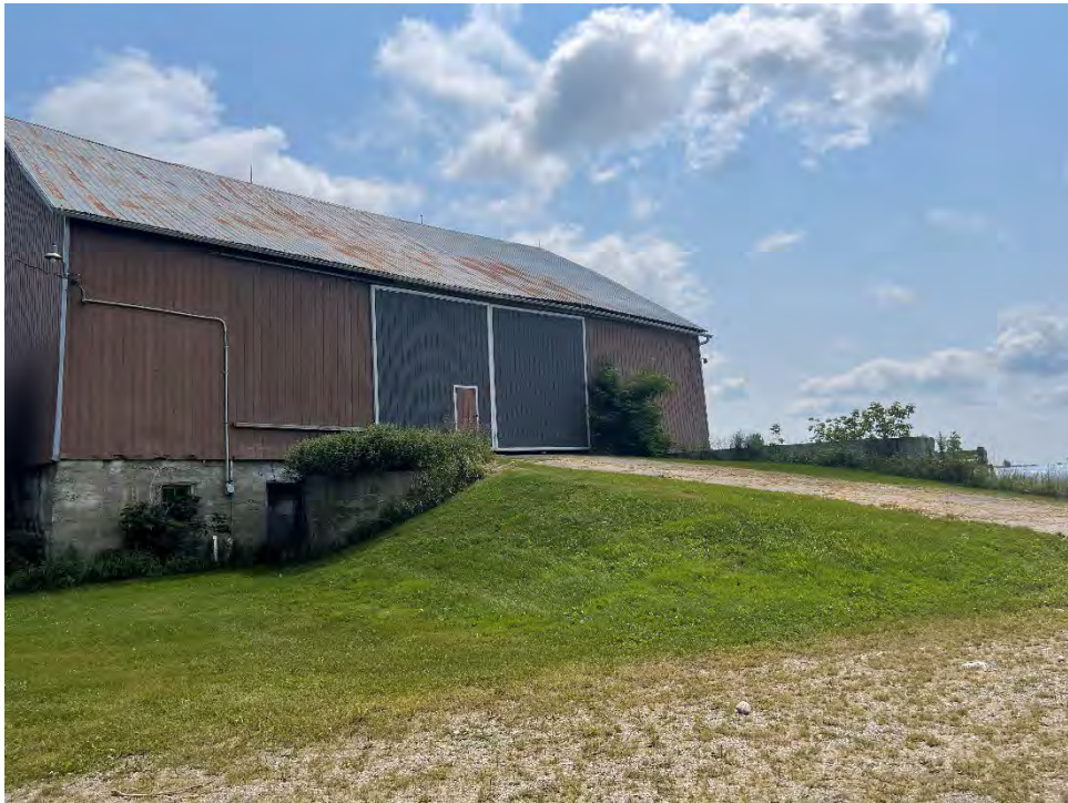
Photograph J9 – Ramp to aboveground level of barn, suspected unknown fill material.
