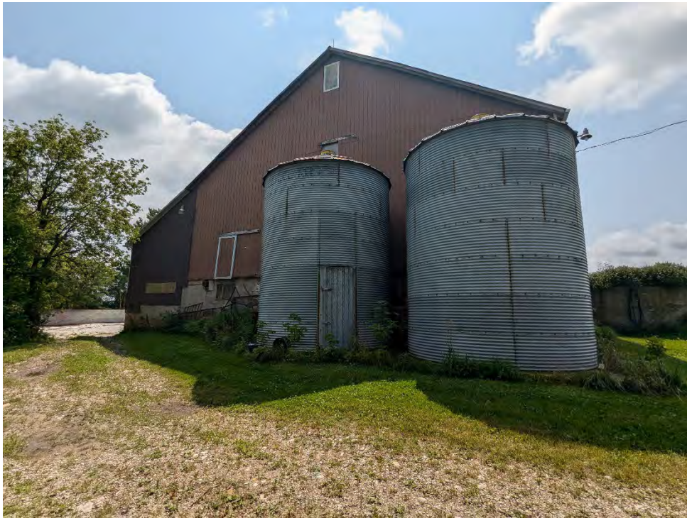
Photograph J15 – Two silos on the north side of the barn, looking south.
