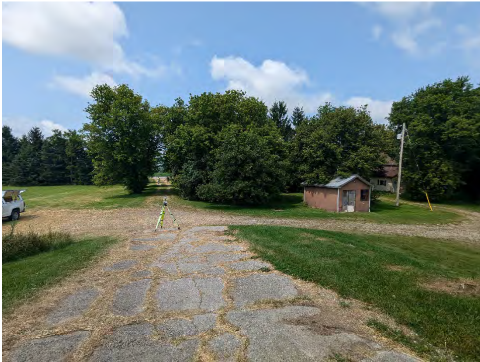
Photograph J19 – Shed west of barn and pole-mounted transformer, looking west.
