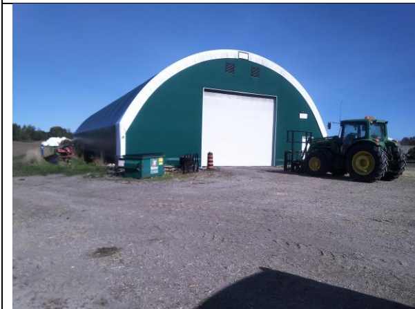
IMAGE 15 OUTBUILDING AND GRAVEL SURFACE
