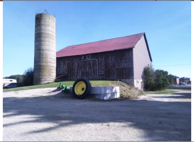
IMAGE 14 BARN AND SILO
