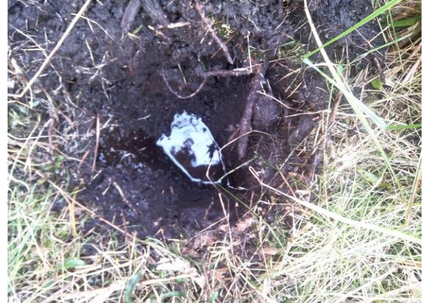
IMAGE 50 WATERLOGGED TEST PIT
