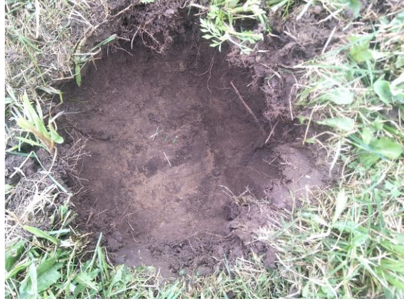
IMAGE 7 COMPLETED TEST PIT
