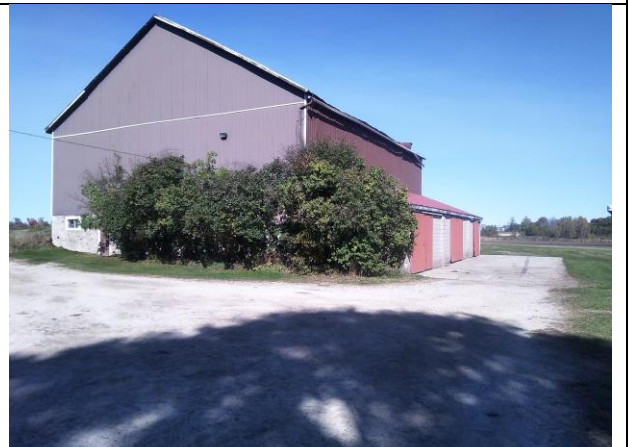
IMAGE 12 BARN AND GRAVEL SURFACE
