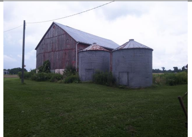
IMAGE 2 BARN, SILOS, AND TEST PIT SURVEY CONDITIONS
