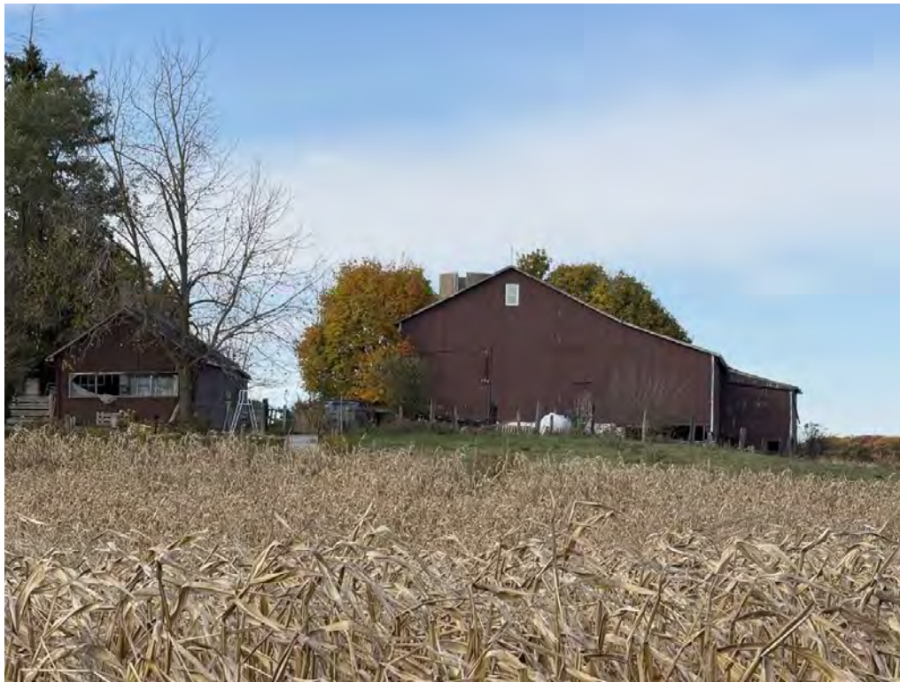
Livestock Barn at 3367 Townline Road
