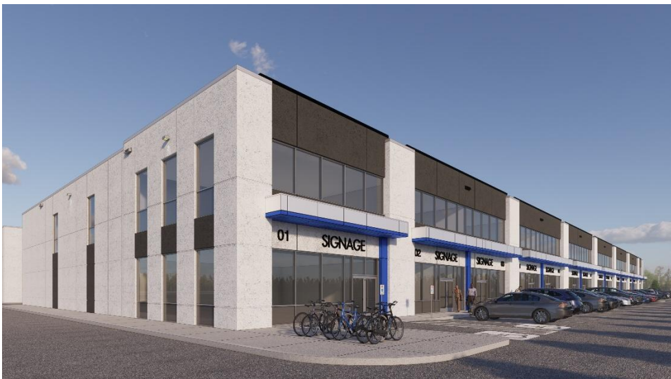
Figure 4: Typical storefront features for industrial condos.
