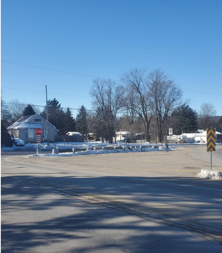
Wellington Road 52 at Ninth Line. Recommended solution includes removal of right turn channel and conversion to all-way stop control.
