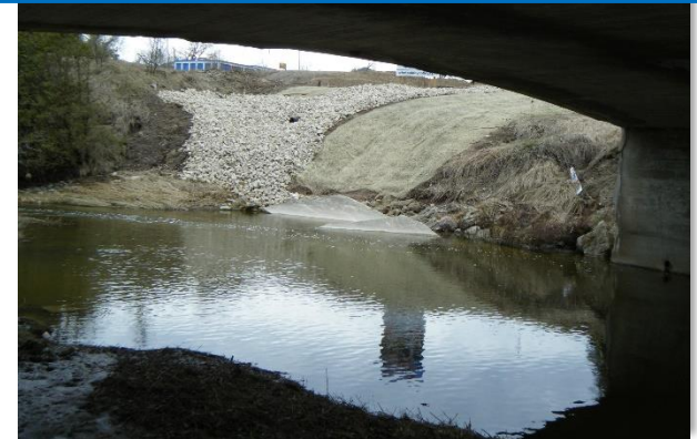
Bank stabilization measures have been put in place to address erosion on the outside meander bend on the south side of the bridge
