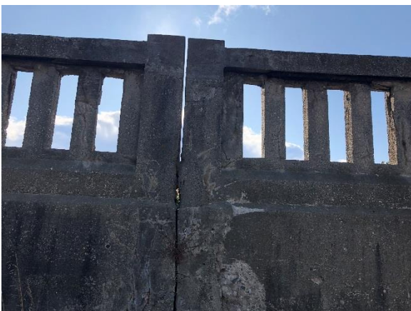
Image 7: View of hand rail, note construction joint between abutment and deck/superstructure
