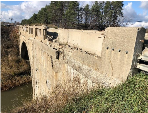
Image 3: Balustrade deterioration detail, looking northwest.
