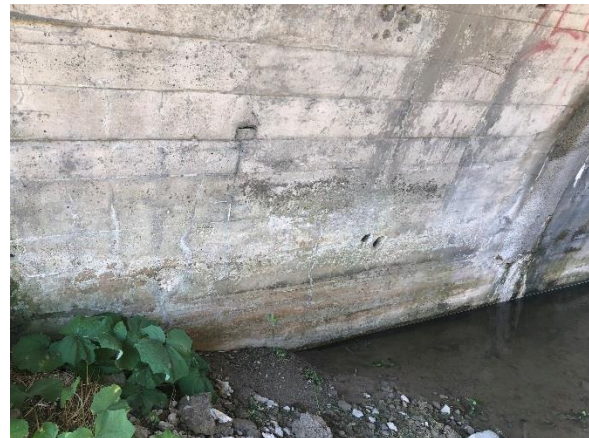
Image 12: Conestogo River Bridge #5, arched concrete wall with formwork detail.
