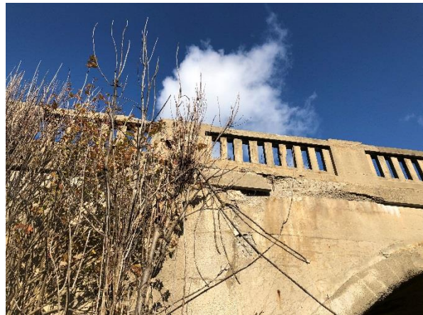
Image 8: Conestogo River Bridge #5, solid spandrel and balustrade railing system.
