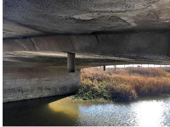
Image 10: View of the underside of the bridge deck, note drainage pipes
