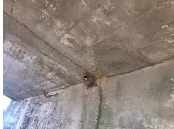
Image 10: View of west abutment and bridge soffit, note the formwork outlines in the concrete used to cast the concrete
