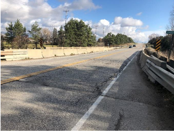
Image 5: Conestogo River Bridge #5, asphalt deck and concrete barrier detail, looking east.
