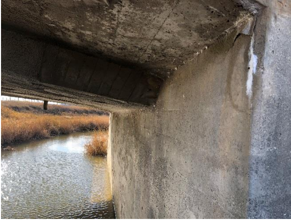
Image 9: Looking north towards west abutment, note concrete accretion on the soffit
