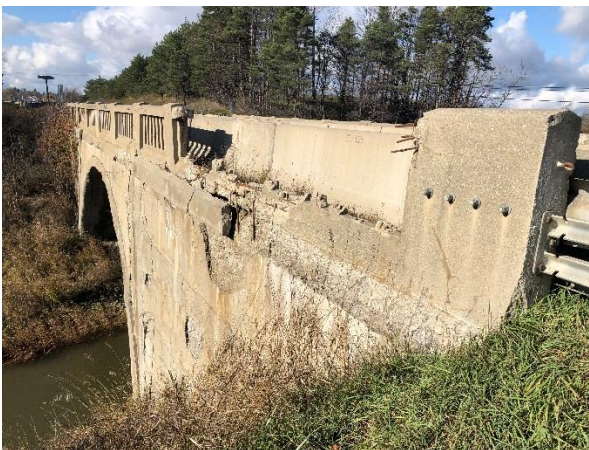
Image 3: Balustrade deterioration detail, looking northwest.
