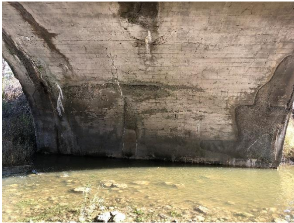
Image 11: Conestogo River Bridge #5, substructure arched concrete with shotcrete repairs.
