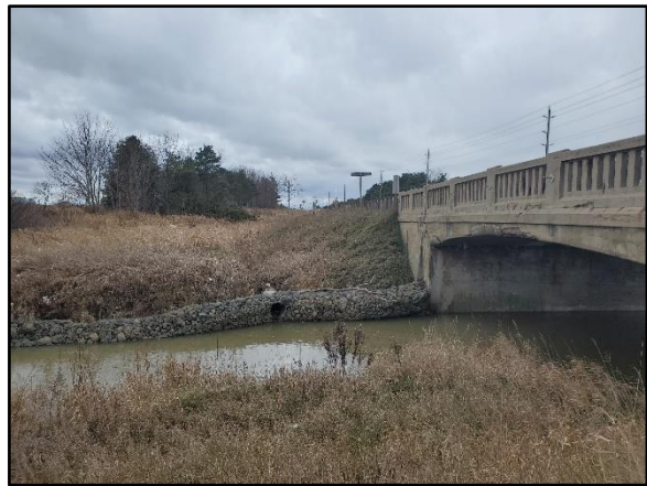
Image 20: Berm, culvert, and ditching disturbance on southwest side of Bridge 3. Photo facing Southwest
