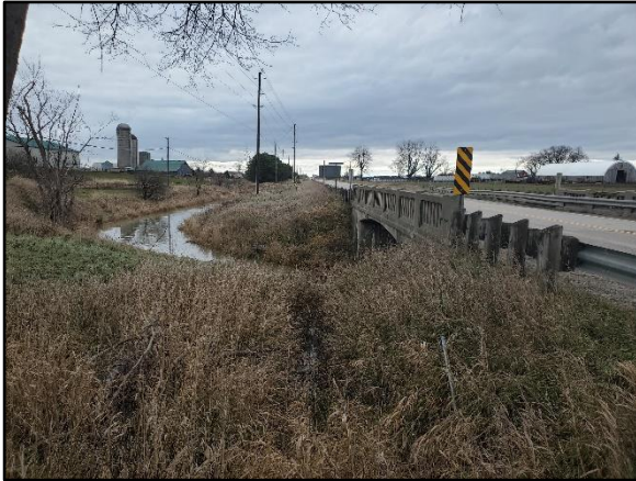
Image 22: Berm and ditching disturbance on northwest and northeast side of Bridge 4. Photo facing Northeast
