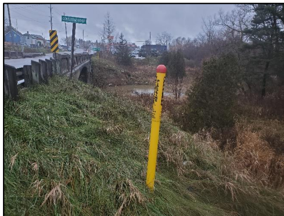
Image 10: Typical indicators of underground utilities and berm of northwest side of Bridge 1. Photo facing Southwest.
