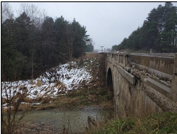
Image 13: Berm and ditching disturbance on southwest side of Bridge 2. Photo facing Southwest
