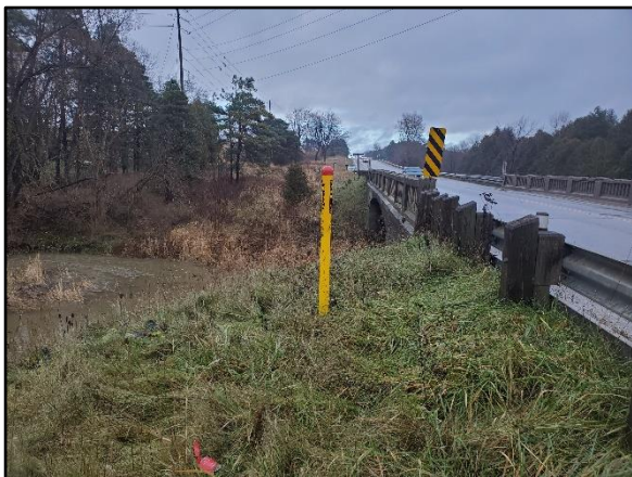
Image 9: Typical indicators of underground utilities. Photo facing Northeast
