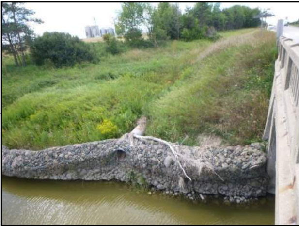
Photo 22: west bank (gabion) and vegetation in the SW quadrant
