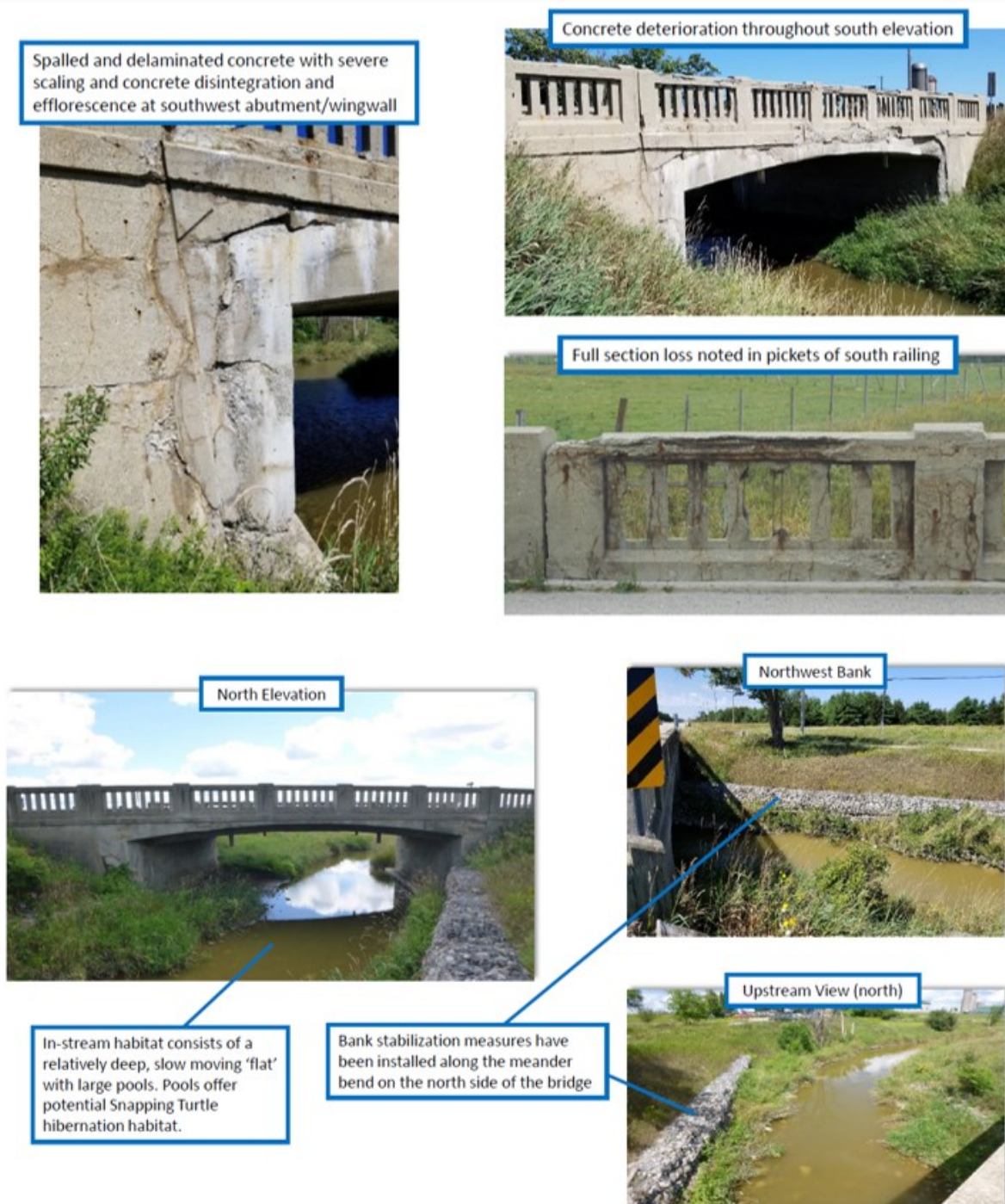
Figure 5-6: Existing Conditions - Structure B109134
