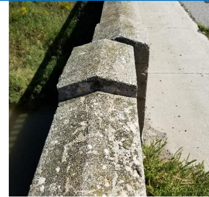
Spalled and delaminated concrete with wide cracks and efflorescence at northwest wingwall
