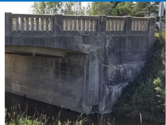
Spalled and delaminated concrete with wide cracks and efflorescence at northwest wingwall
