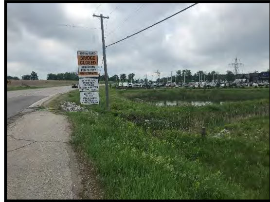
Image 18: Disturbed Lands – Ditch and Drainage (May 31, 2018; Facing South)
