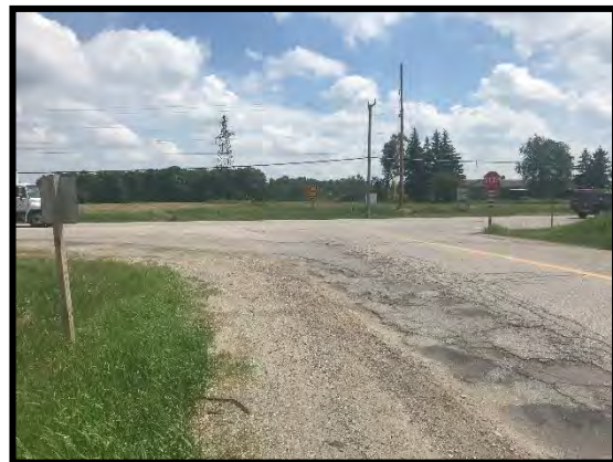
Image 64: Disturbed Lands – Roadway (May 31, 2018; Facing East)
